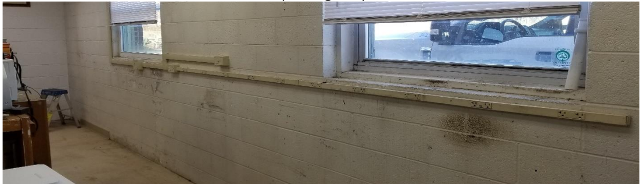
Office painting completed
