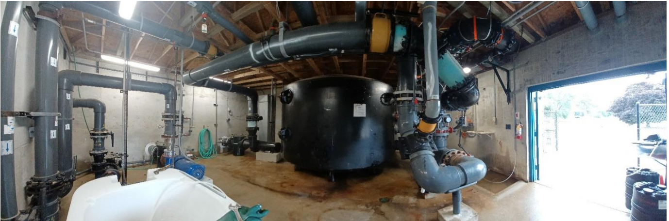
FILTER/PIPING REMOVAL COMPLETED
