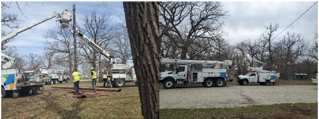
UTILITY POLES – CITY PARK
