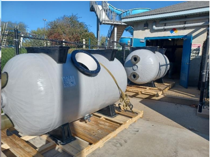
NEW FILTER/PIPING INSTALLATION
