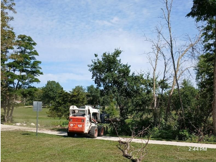
POOL TREE REMOVAL
