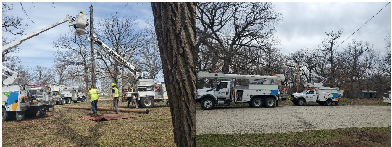
UTILITY POLES – CITY PARK
