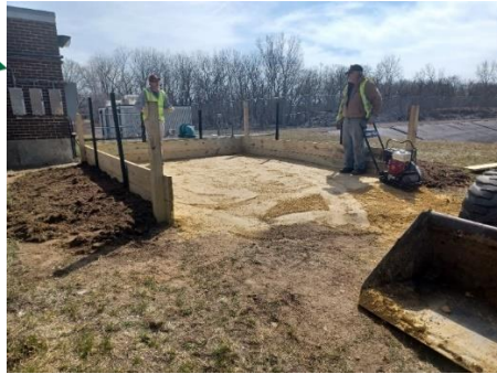
GRAVEL BED CONSTRUCTION COMPLETED
