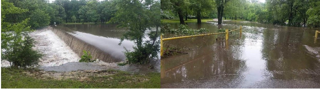
FLOODING AT CITY PARK
