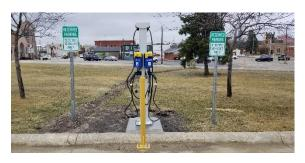
The car charging station is up and running. This Level II station is located on the northwest corner of the library parking lot. Users will need to download the app to sign up for a free account. The Electric Vehicle Charging Station was paid for by the Iowa Department of Transportation Volkswagen Settlement Environmental Mitigation Trust program. The total cost for the unit and installation was \$13,858. The amount to be reimbursed through the grant is \$12,472.
