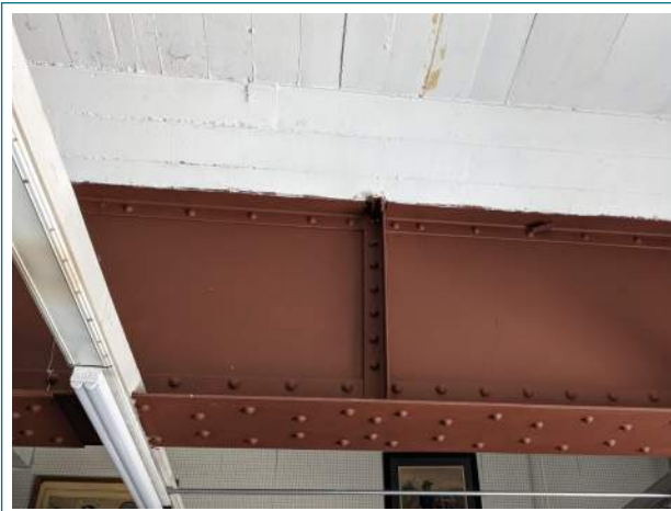
WIDE FLANGE BEAM STRUCTURE P-11
