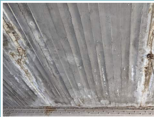
BOARD FORMED CONCRETE P-17
