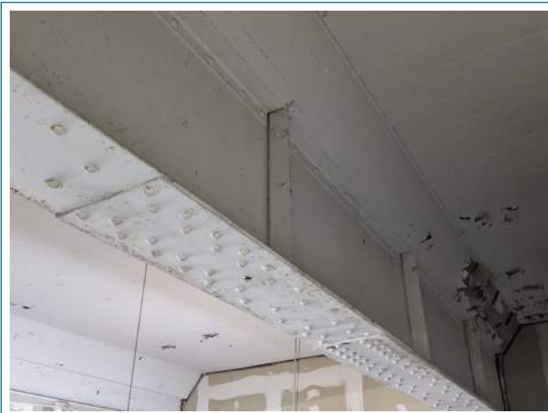
WIDE FLANGE BEAM STRUCTURE P-10
