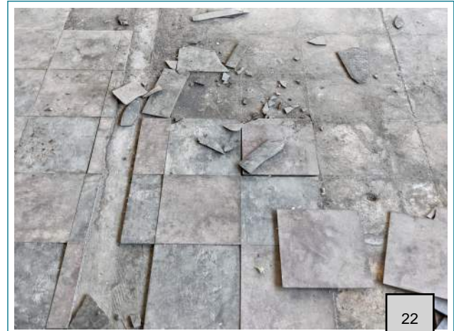
POTENTIAL ASBESTOS CONTAINING TILE P-18
