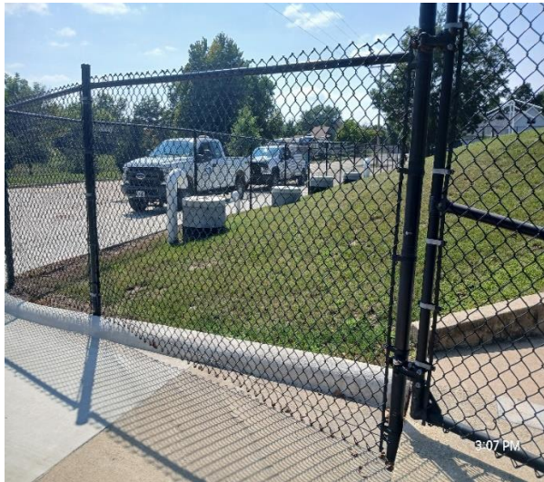
GAS SHUT OFF
