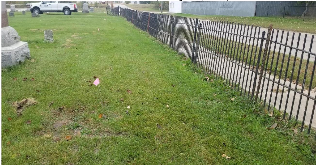
Front Oakdale Cemetery fencing held up with t-posts
