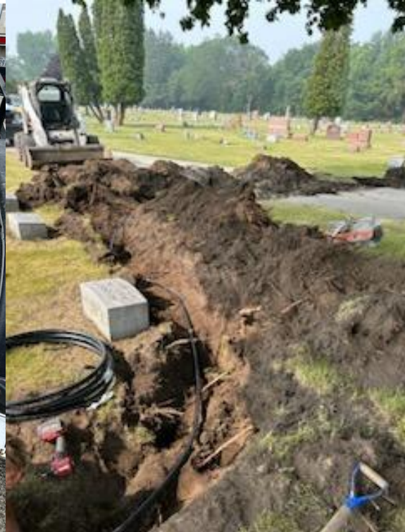
WATER LINE REPAIR
