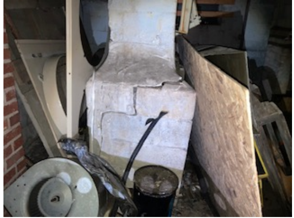
Chimney no longer in use.
