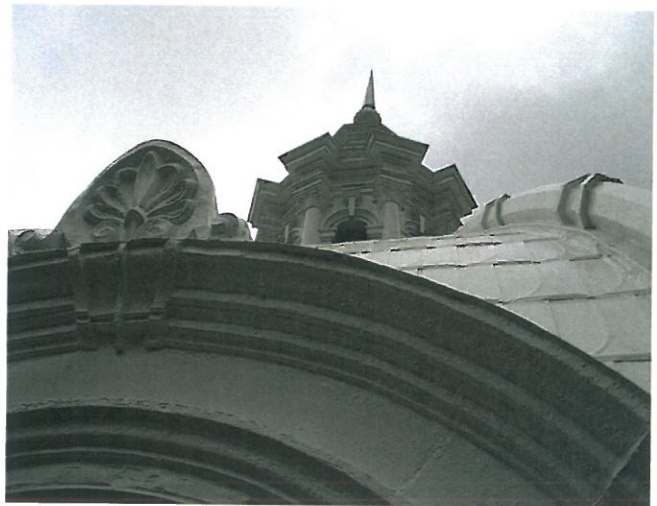
Dome Restoration Detail
