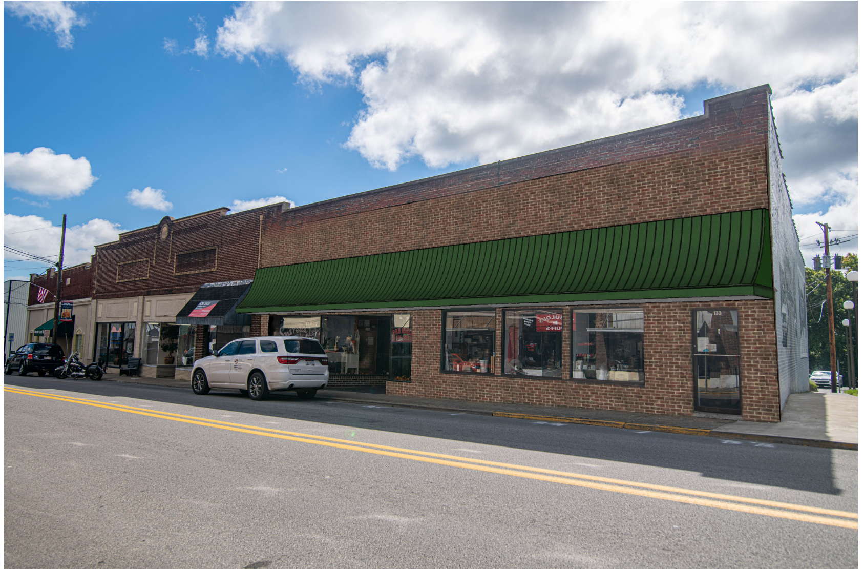
133 Main Street New fabric canopy. Brick at sidewalk level restored.
