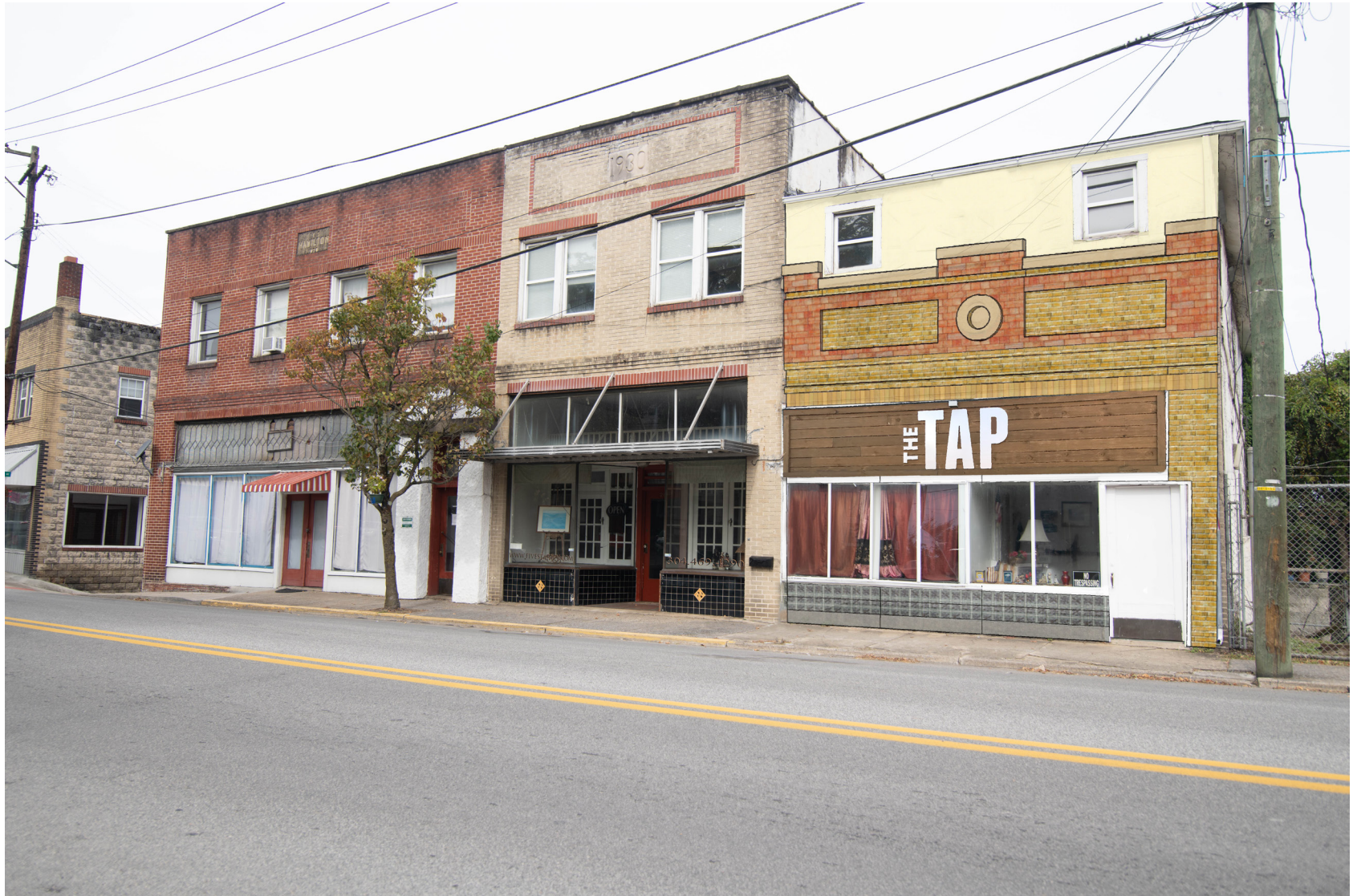
201 Main Street Clean original brick facade and paint upper addition. New modern signage.
