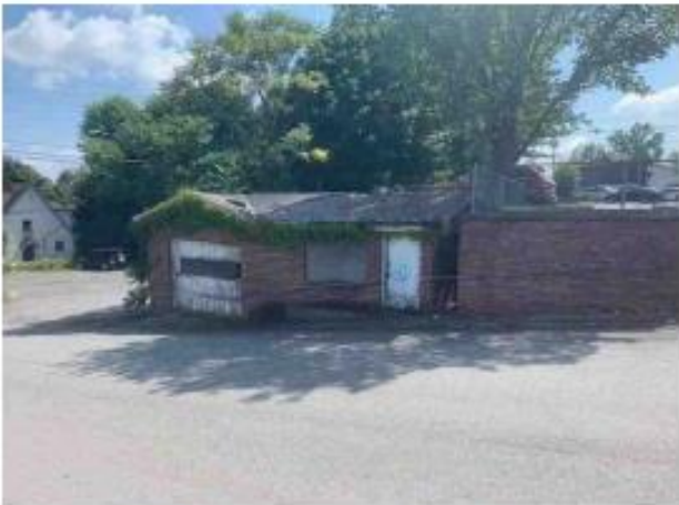
Old Garage Needs Torn Down
