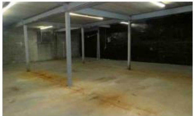
Unfinished Basement Area
