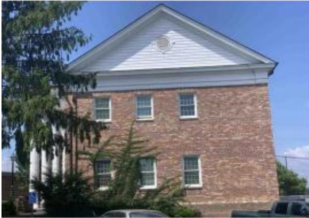
Right Side View of Building
