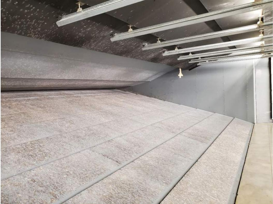
Photograph 19: Hero Center ammunition collection baffles
