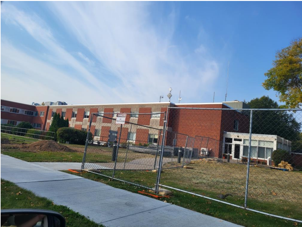
Looking SW from Columbus Ave. N. at the location of the proposed building addition.
