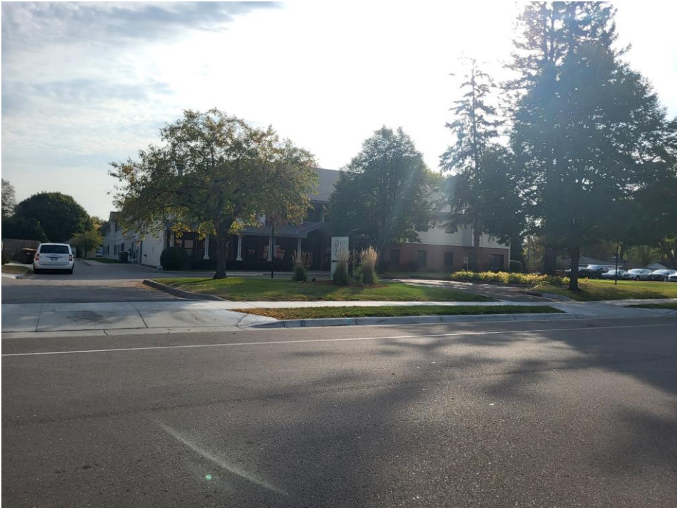
Looking at the east side of Columbus Ave. N. at Queens Court building which is across the street from the proposed addition.
