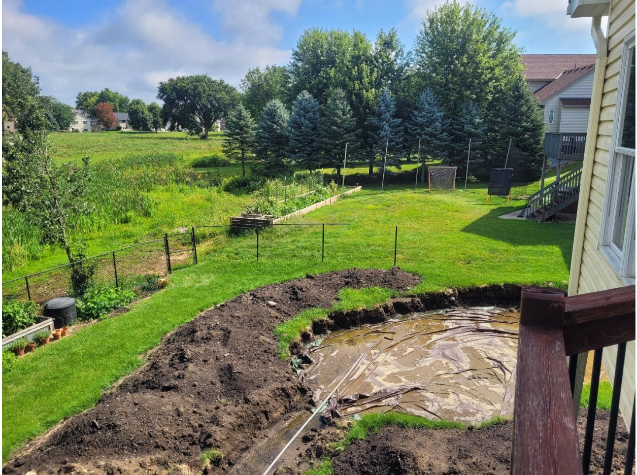
Figure 12. Looking east from deck. Note the current excavated area is larger than the actual pool itself, as well as the slope on the side of the house.
