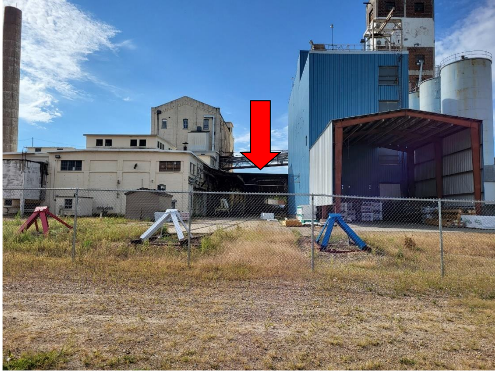
View of Canopy Area from Main St. W. (middle of the photo) – Other stored items in this photo must be moved to storage area under canopy.
