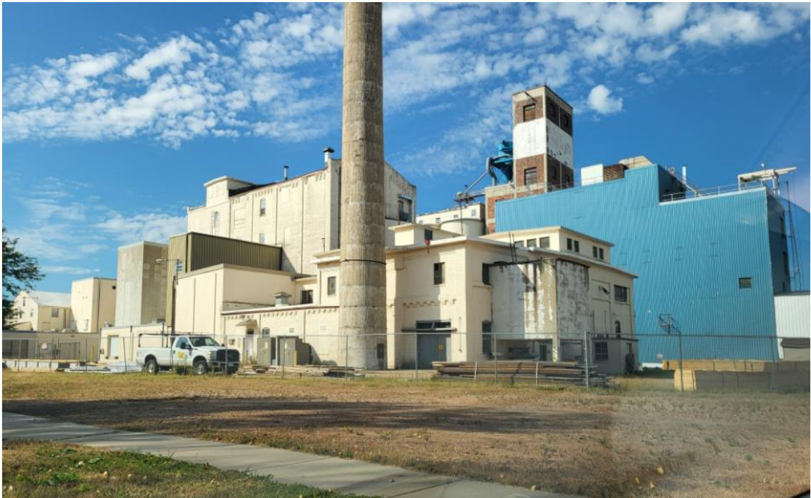
Looking at site from 2 nd Ave. SW (these exterior storage items must be removed and fence revised to only enclose storage or other areas not yet being rented/occupied).
