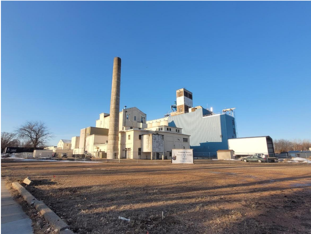
Picture of the Mill Looking Southwest from 2 nd Ave SW
