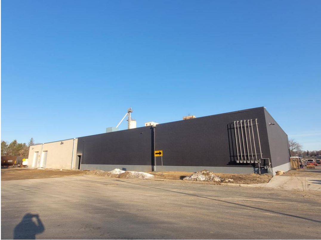
Back of 2 If By Sea Tactical Shooting Range Looking North from the City ROW/2 nd Ave SW
