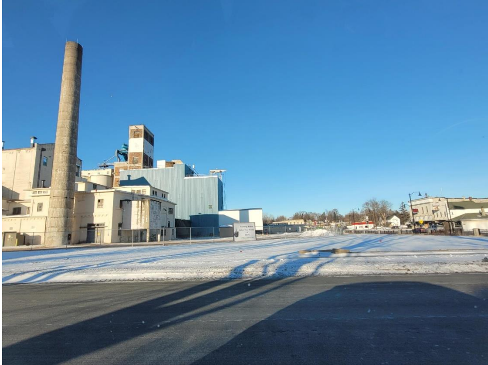
Looking West from 2 nd Ave SW
