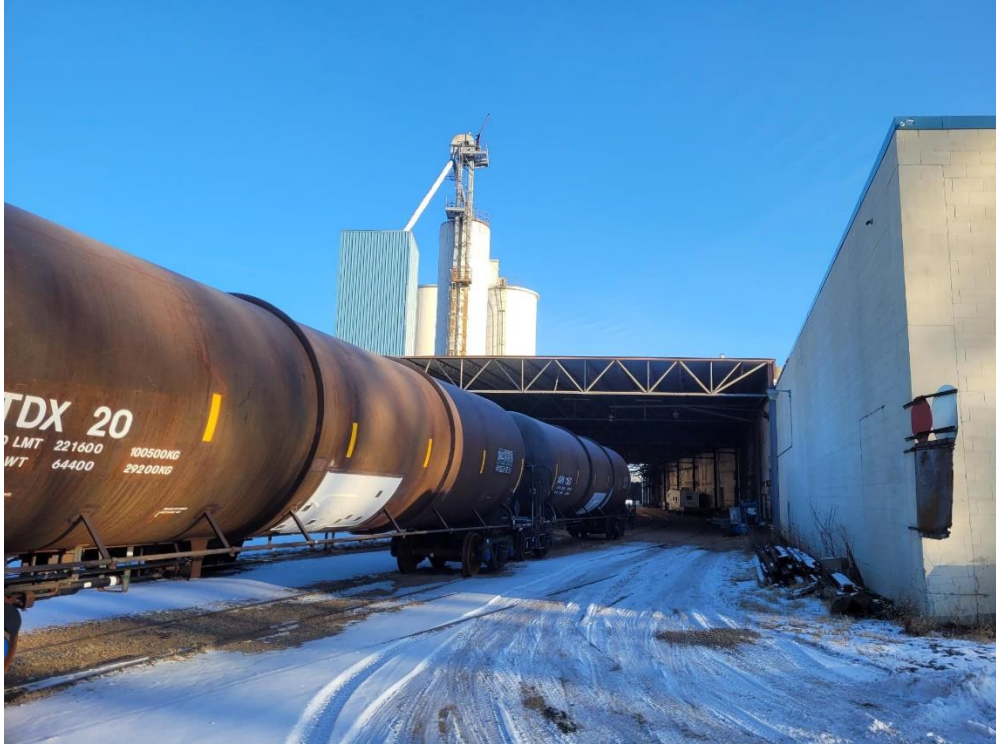
Looking North on the Rail Spur Towards the Southside of the Canopy Storage Area
