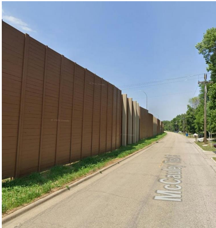
Example of MnDOT Noise Wall Appearance (posts can be inside or outside)
