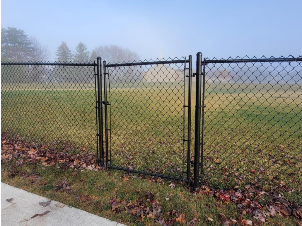
Existing Fence Gate
