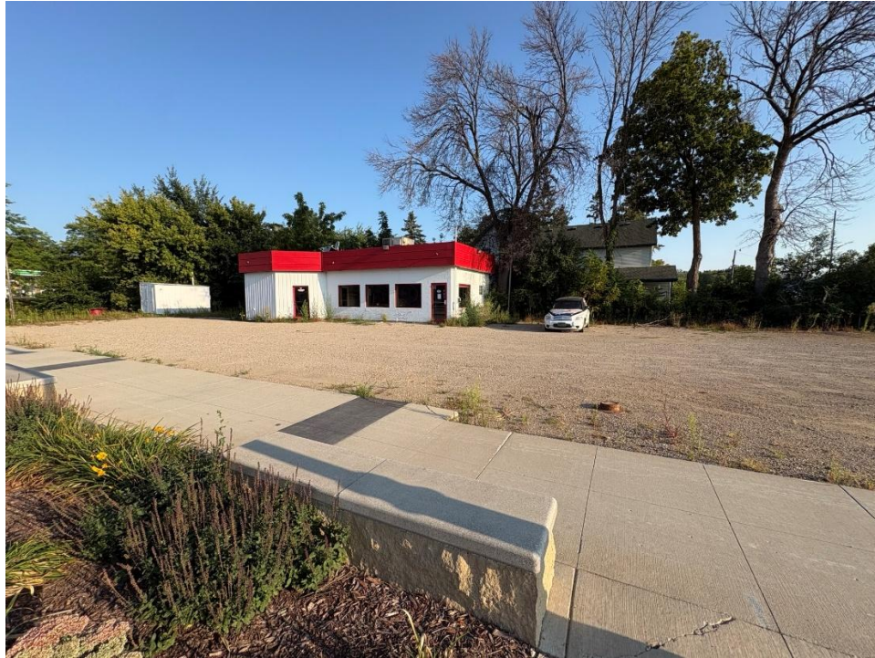
Looking north at the site
