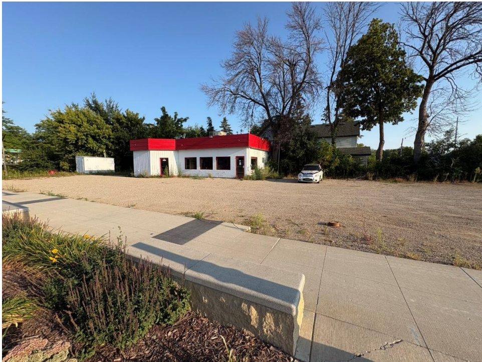
Looking north at the site
