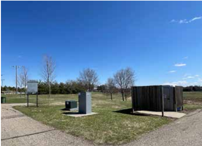
Restroom Enclosure & Electrical Cabinets
