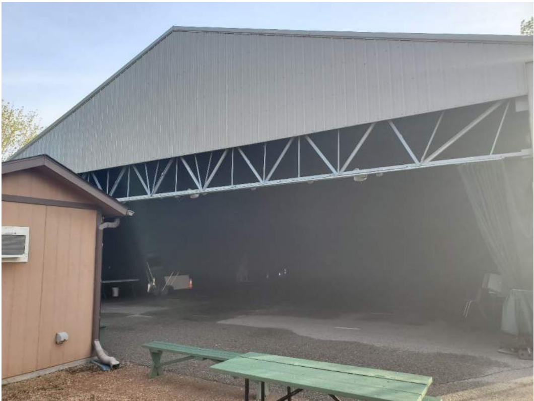
Photograph 15: Tactical gun range and warming hut
