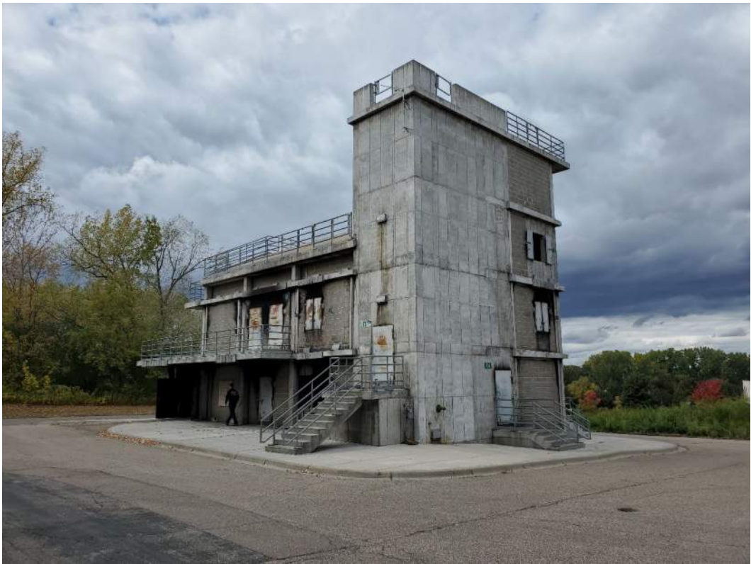
Photograph 24: South Metro tactical fire training tower
