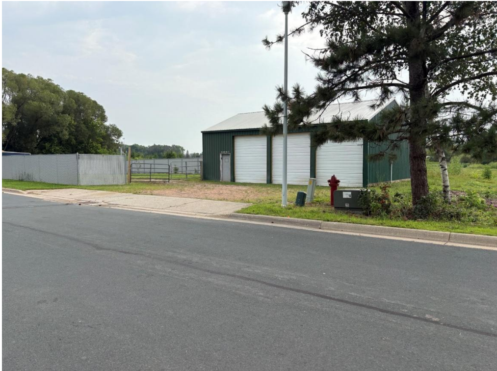
Garage currently located at 903 1 st Ave NW
