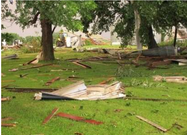
Figure 13. Damage from Tornado in Belle Plaine, MN, July 15, 2019
