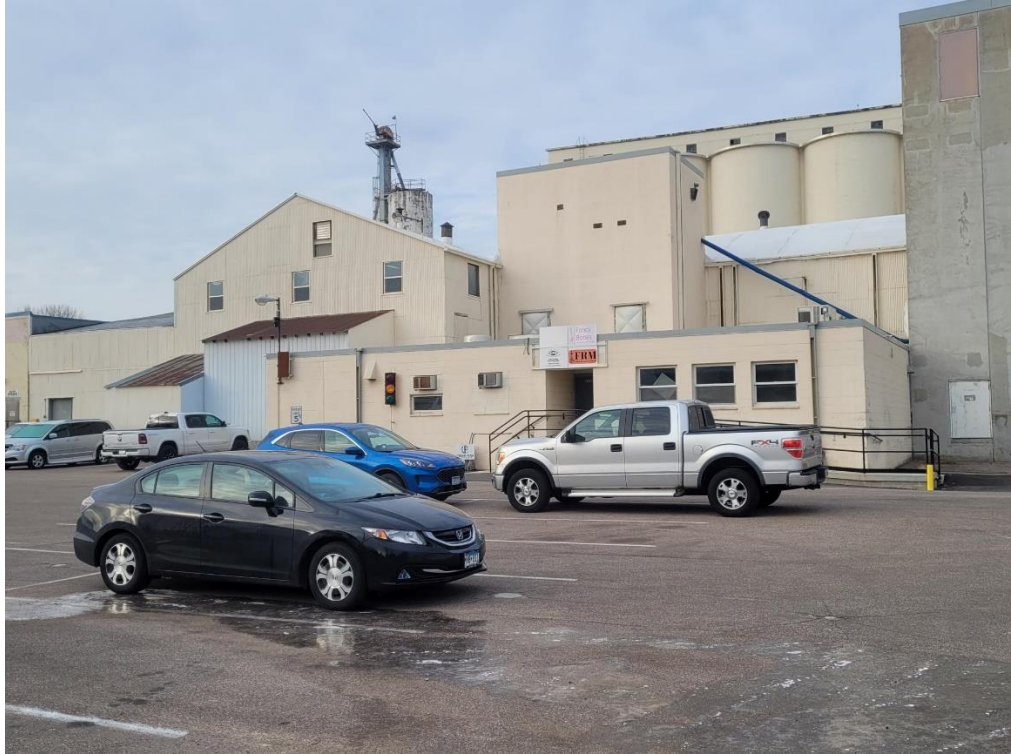
Looking West Towards the Office Entrance
