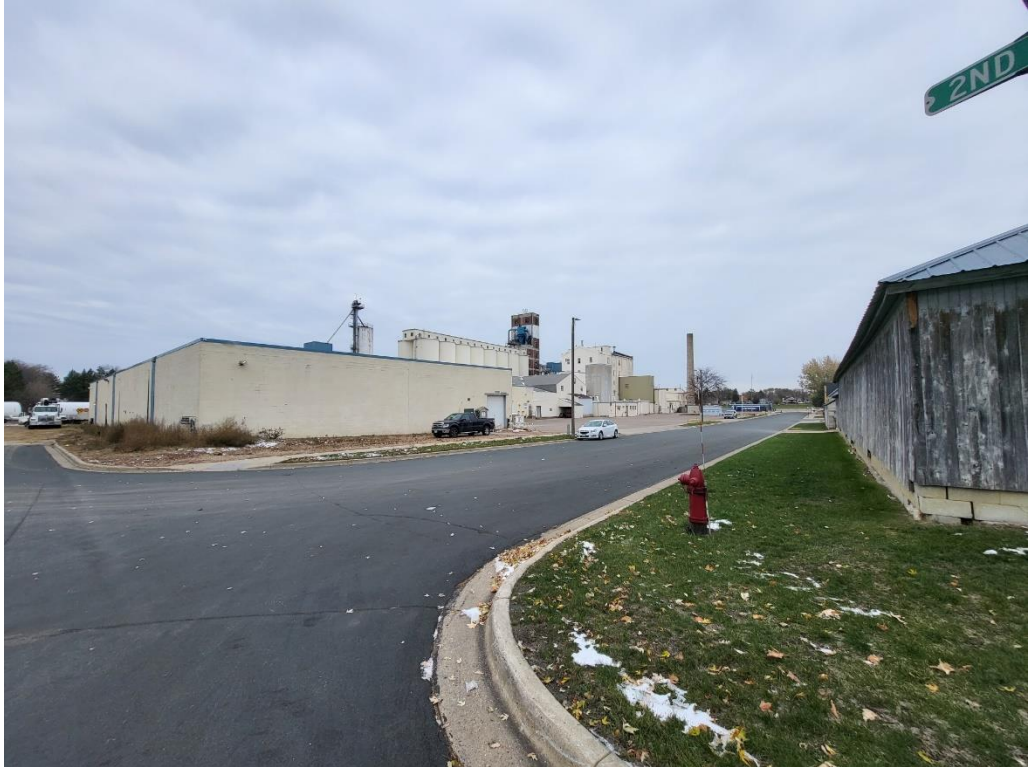
Looking NW towards previously approved Indoor Firing Range – Main Entrance will be on the east elevation of the building along with 2 ADA Parking Spaces
