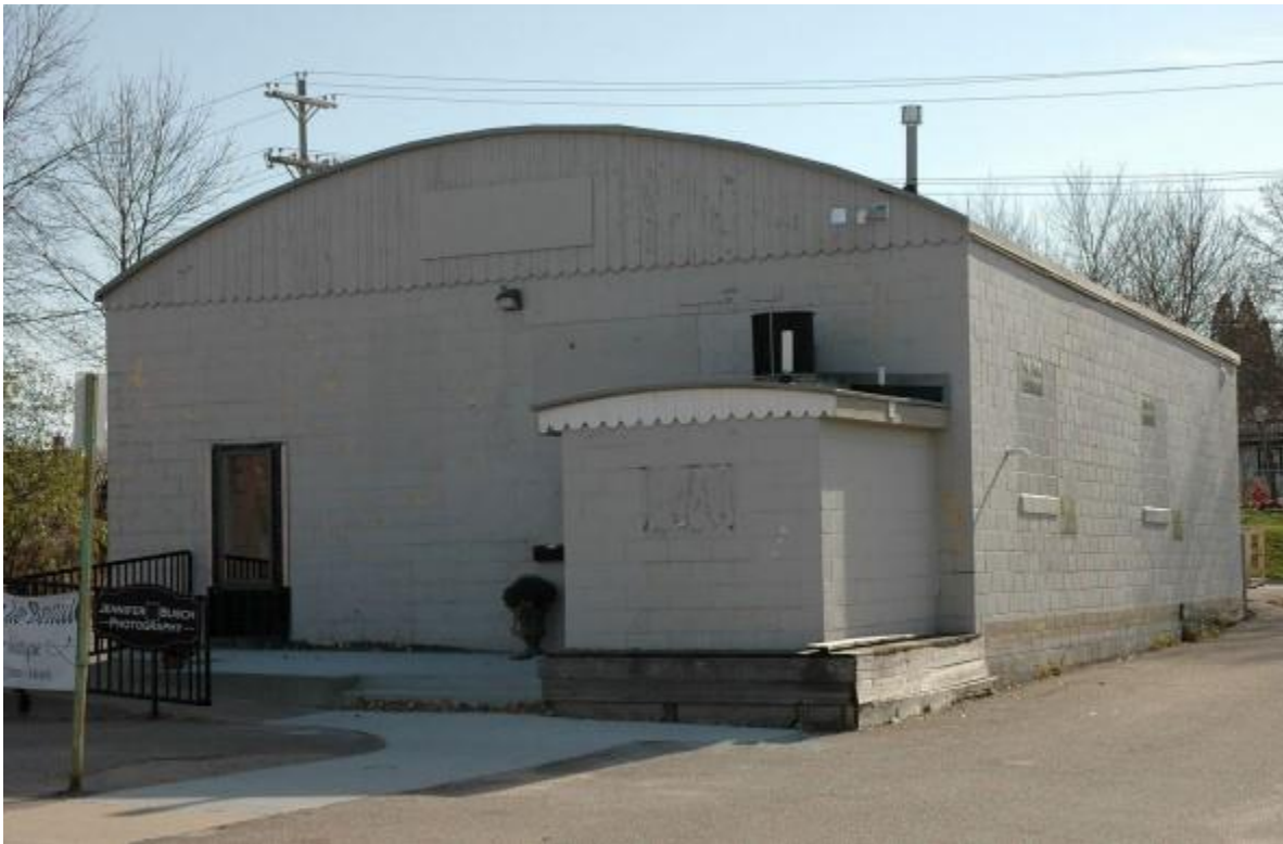
126 Main St W - Cement Block Cladding
