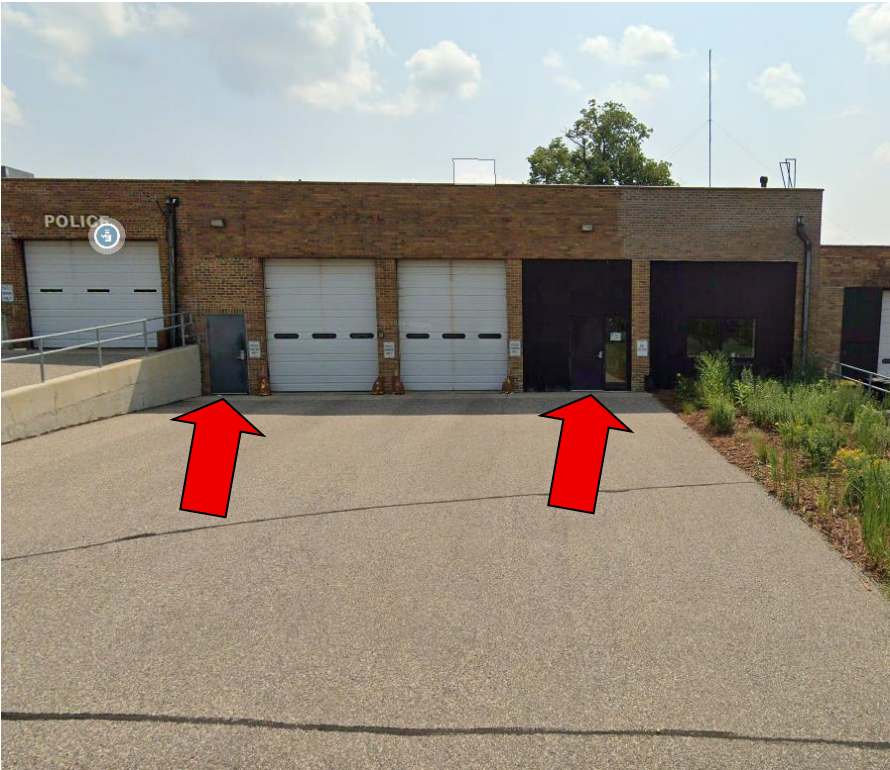
Entrance to Precinct in former Park Department Office Area
