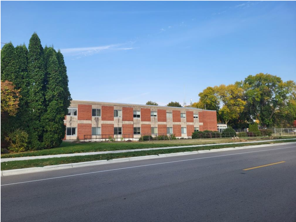
Looking NW from Columbus Ave. N. at the location of proposed building addition.
