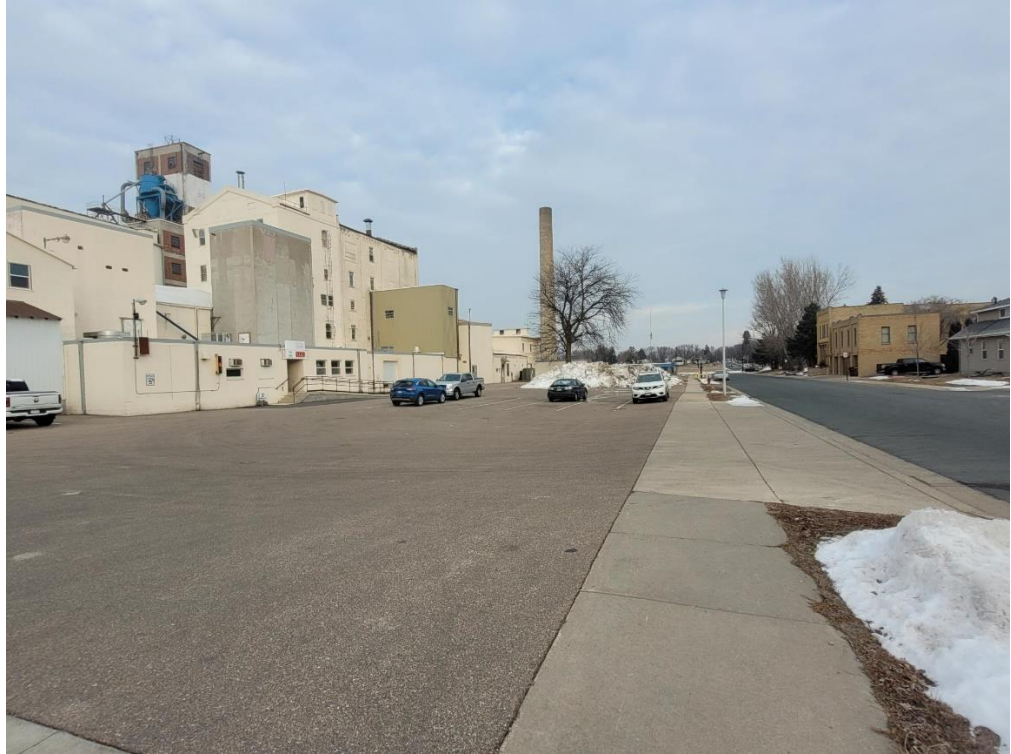
Looking North Along 2 nd Ave SW
