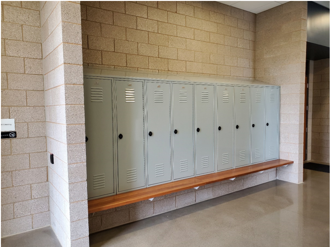
Photograph 21: Hero Center hall storage
