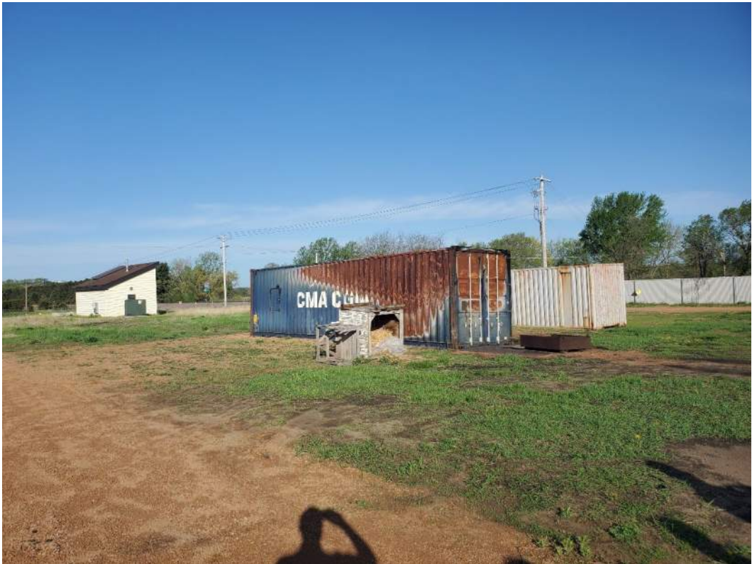
Photograph 18: Class A training Connex boxes
