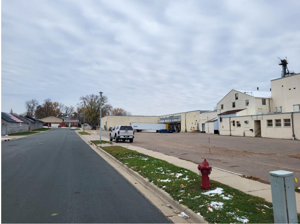
Looking South along 2 nd Ave. SW – parking area is this paved parking area.
