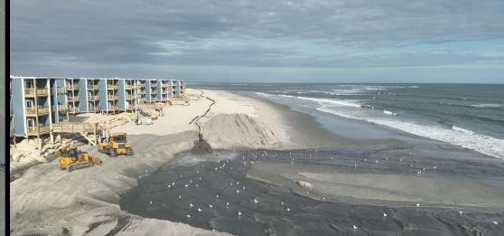
VERTICAL DATUM NAVDRA. THE CONTRACTOR SHALL BE RESPONSIBLE FOR ESTABLISHING HORIZONTAL AND VERTICAL CONTROL PROR TO PLACEMENT OF DREDGED MATERIAL IN THE DESIGNATED PLACEMENT AREA.
