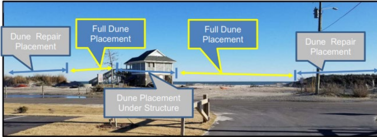
Figure 1: Dune Material Placement (photo taken February 3, 2021).
