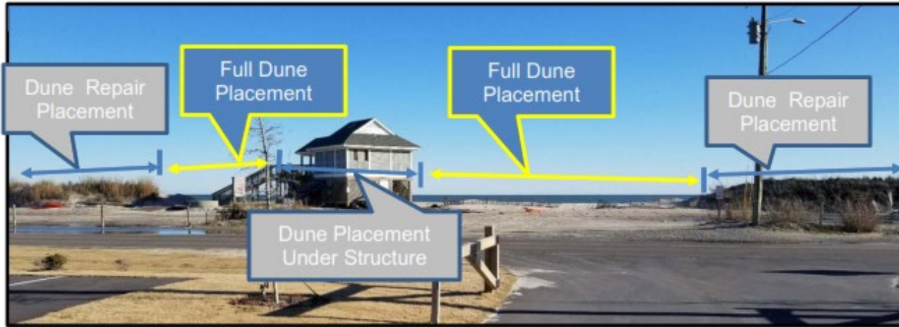
Figure 1: Dune Material Placement (photo taken February 3, 2021).
