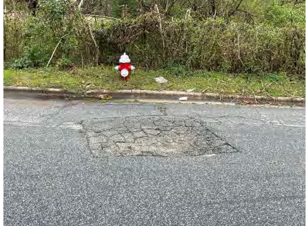
High Severity Patch
