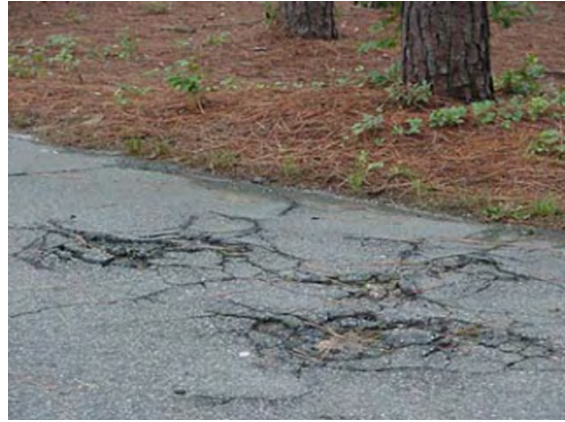
High Severity Roughness
