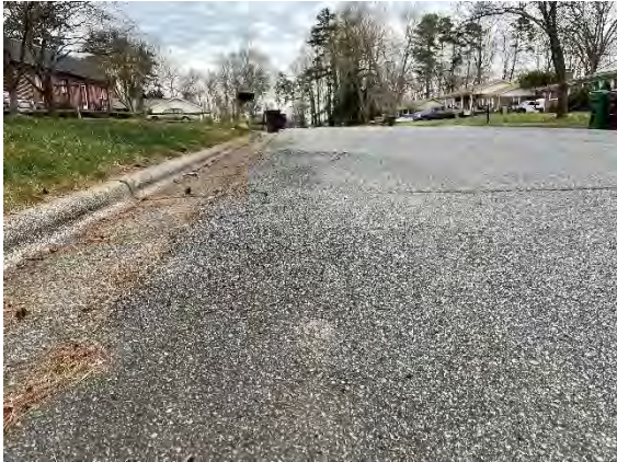
Medium Severity Roughness
