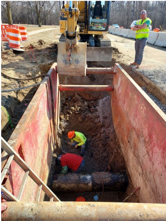
Water Main Work at 10 Mile/Wixom
