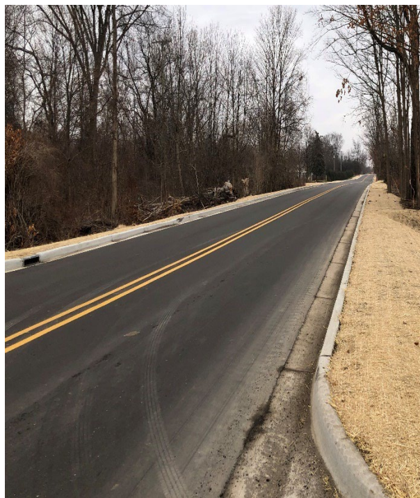
12 Mile Rd - After
