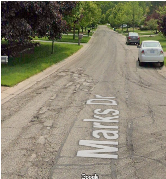
Marks Drive – Before
