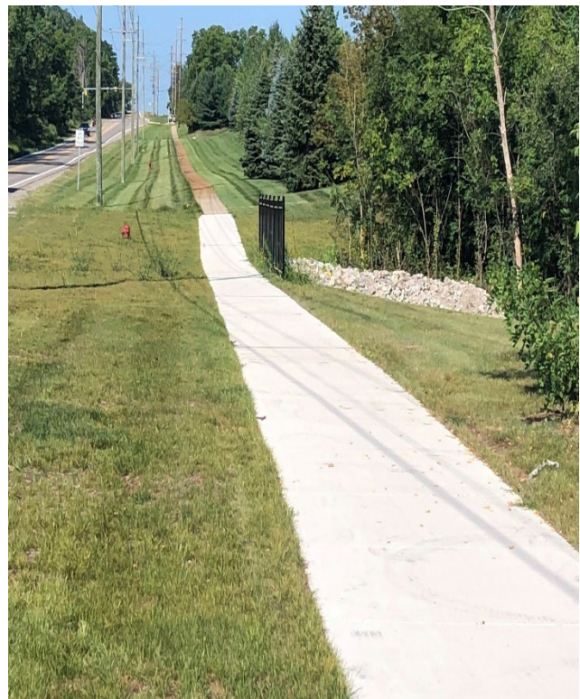
Sidewalk Gap Infill & Culvert Extension
