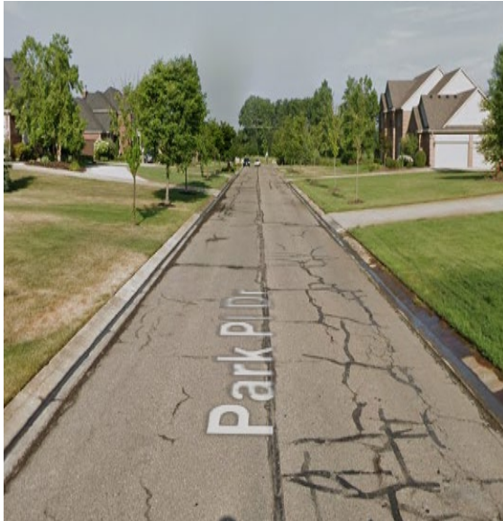
Park Place Drive – Before
