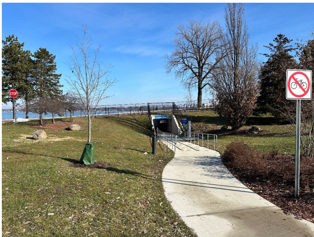
After – Park side (south)
