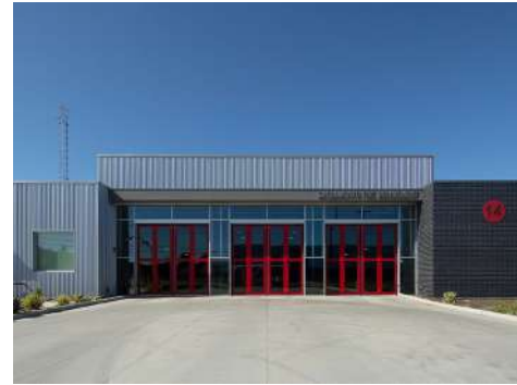
SACRAMENTO, CA FIRE STATION NO. 14
