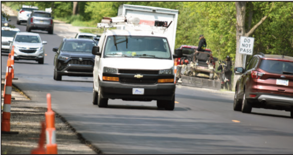
A recently completed preservation overlay project.
