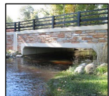
Figure 4: Three-sided box bridge
