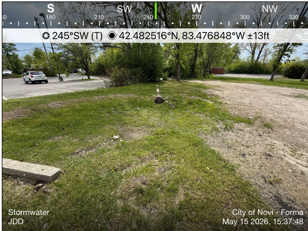
Overview of the stormwater pipe/area on-site
