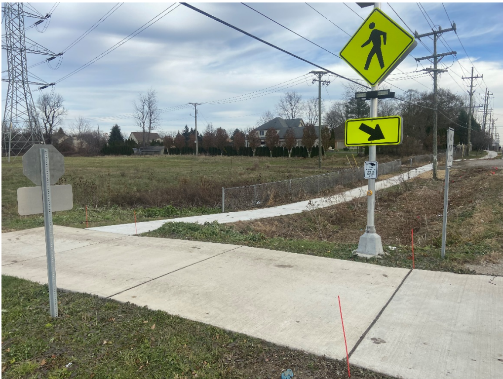
After – At the ITC Corridor, looking east
