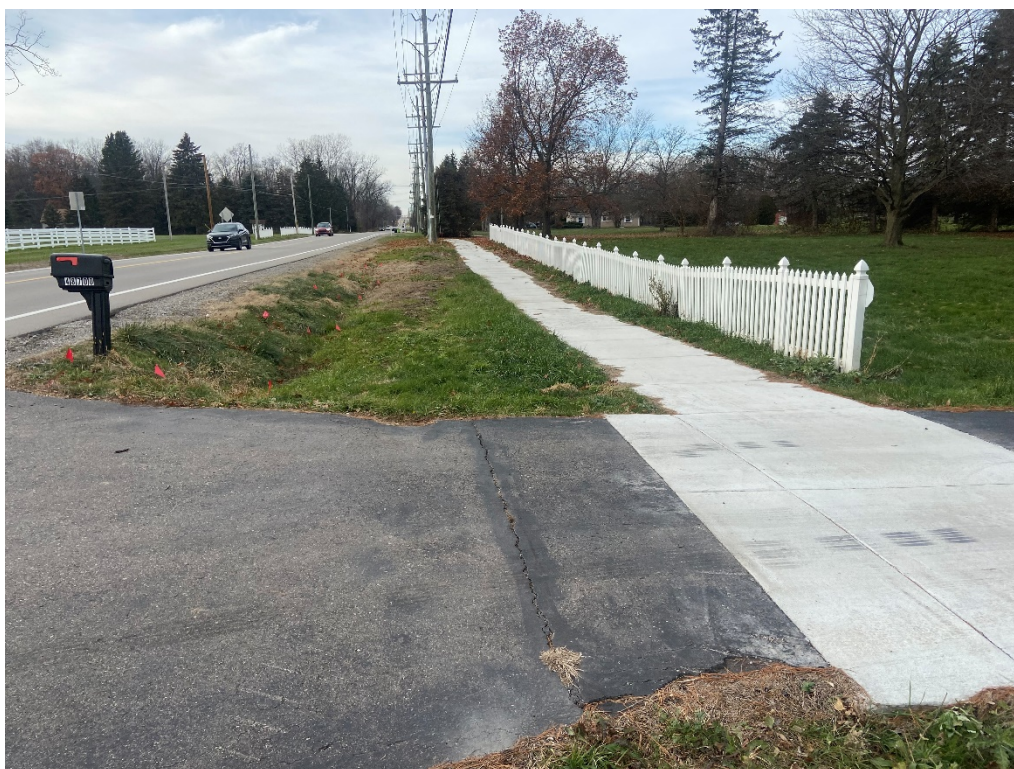
After – West of the ITC Corridor, looking west
