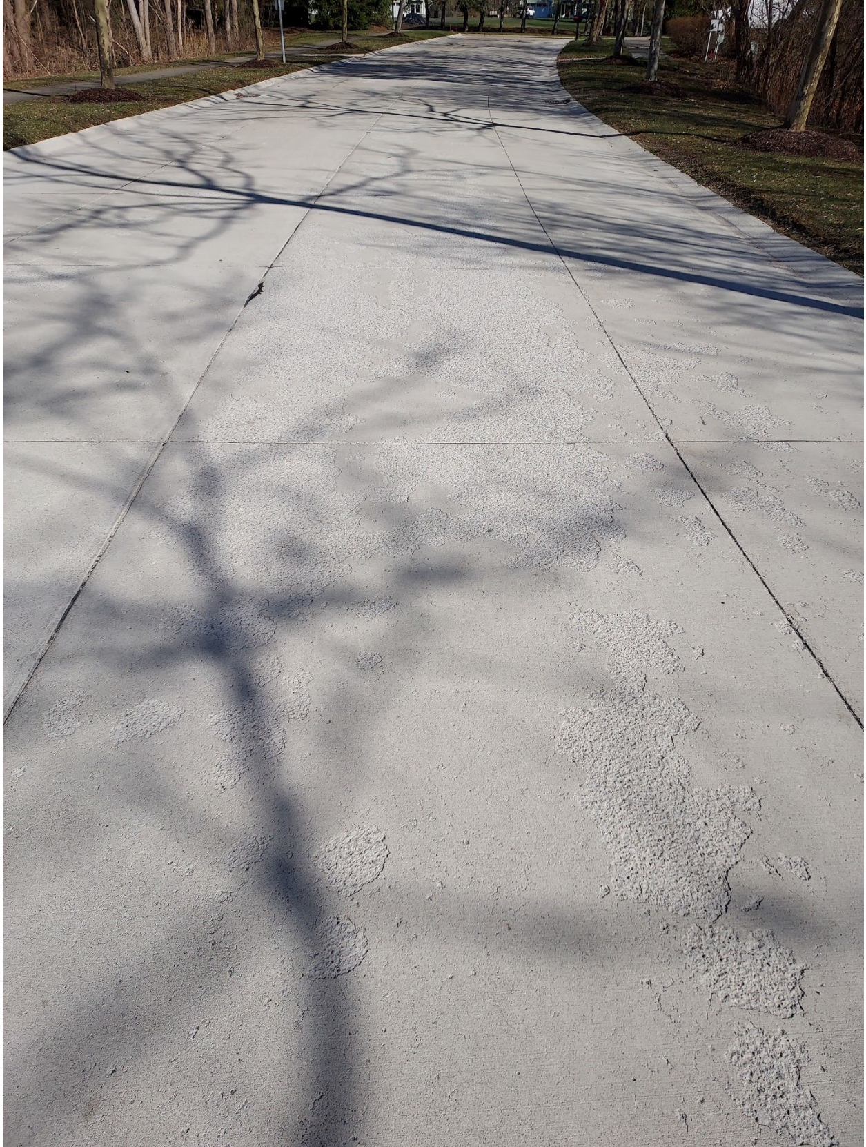
Example 2 – Laramie Drive (Walden Woods II) – South of 11 Mile
