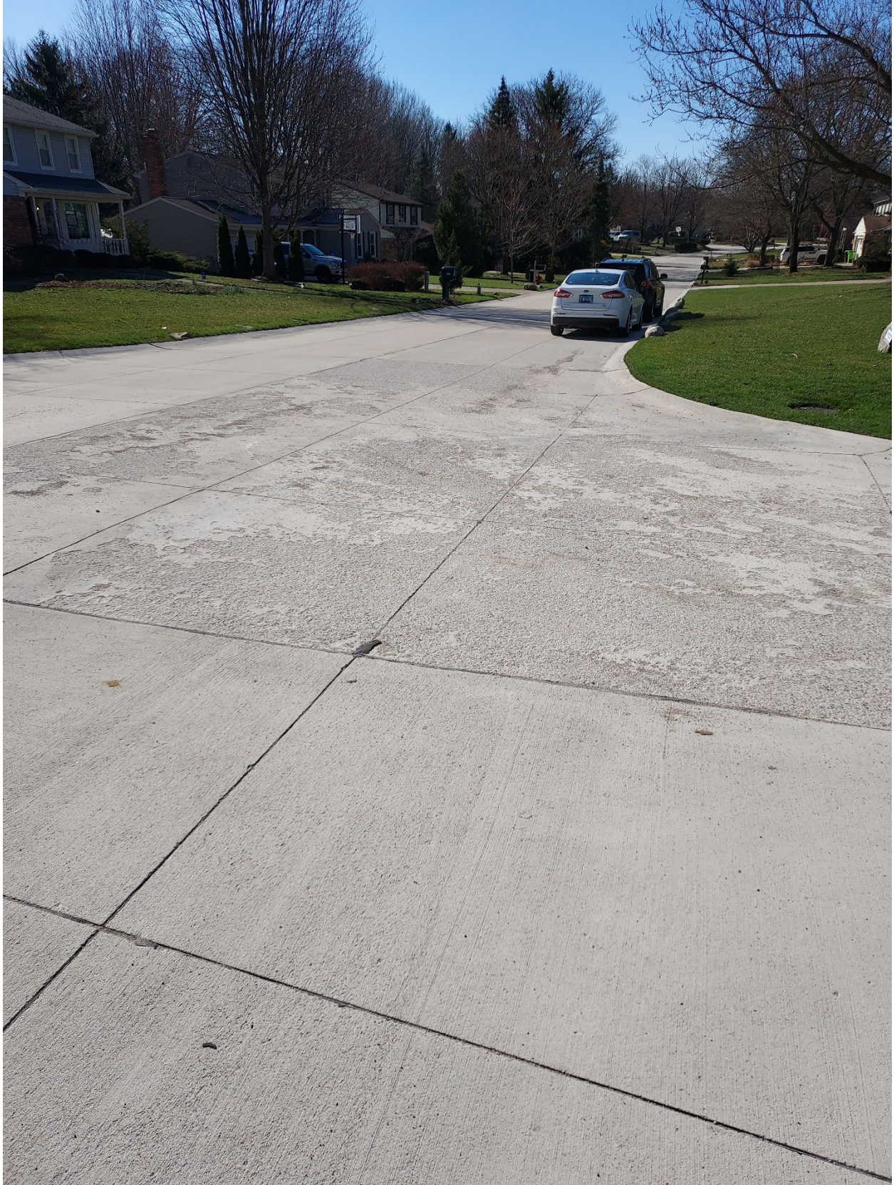
Example 4 – Cumberland Drive (North Hills Estates) – at Ironside Court
