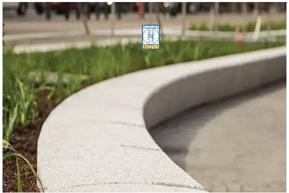
Seatwall 15"W x 18"H Colored concrete, Medium Gray
